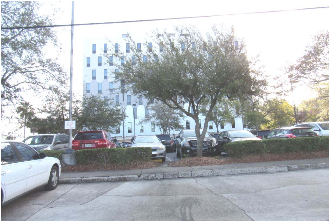
View of building from May Street
